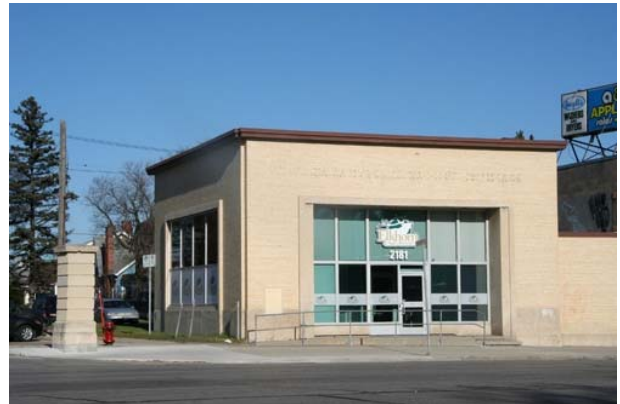
Former Canadian Imperial Bank of Commerce, 2181 Portage Avenue, Winnipeg
