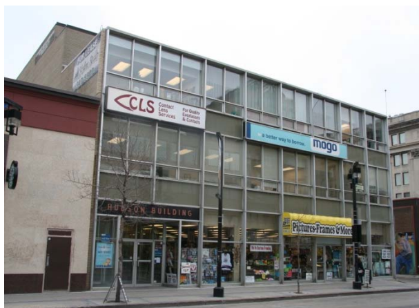
Hudson Building, 1959, 414 Graham Avenue, Winnipeg
