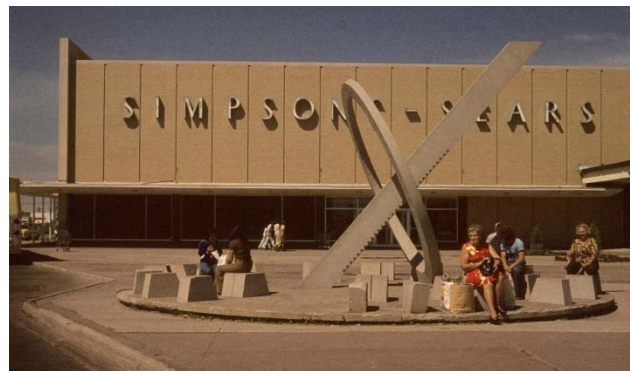
Polo Park Shopping Centre, Winnipeg, Green, Blankstein and Russell, 1958 (historic photos; building massively altered)
