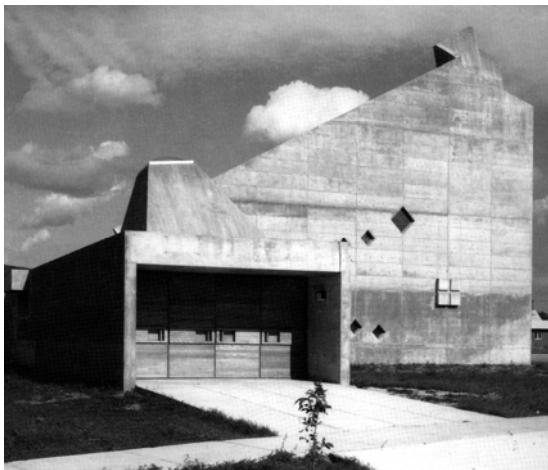
Blessed Sacrament Roman Catholic Church, Etienne Gaboury, 1966. Wabasha Street at Harold Avenue, Winnipeg (Transcona)
