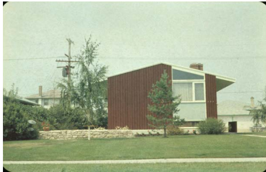
Waisman Residence, Winnipeg. Waisman, Ross & Associates.
