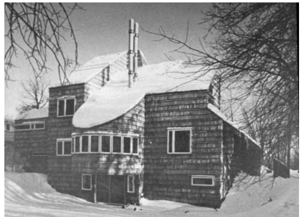
Gaboury Residence, St. Boniface, Gaboury, Lussier & Sigurdson, 1968
