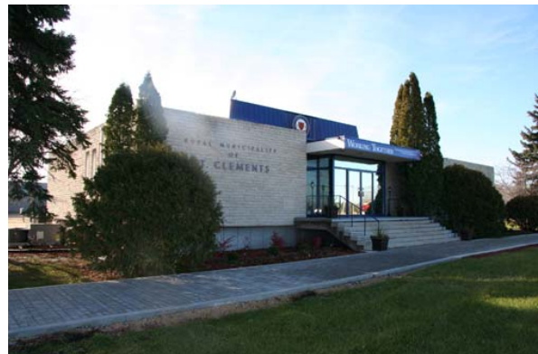
R.M. of St Clements Municipal Building, Hans Peter-Langes, 1968
