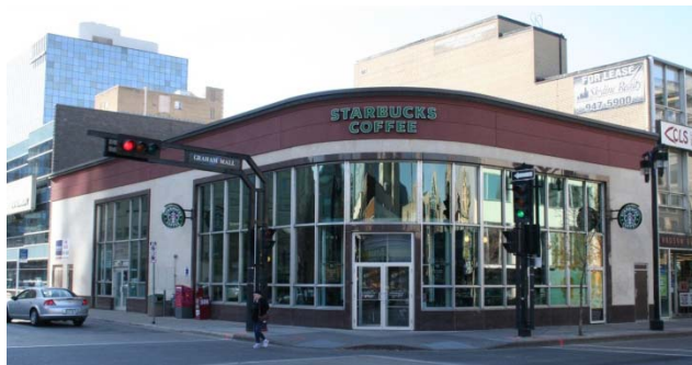
Former Canadian Imperial Bank of Commerce, 1954. 412 Graham Avenue, Winnipeg
