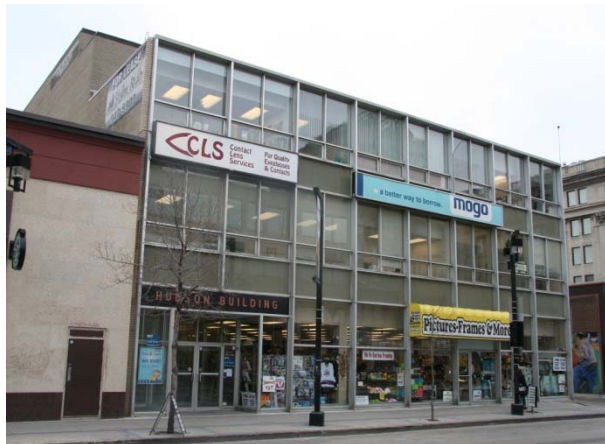
Hudson Building, 1959, 414 Graham Avenue, Winnipeg
