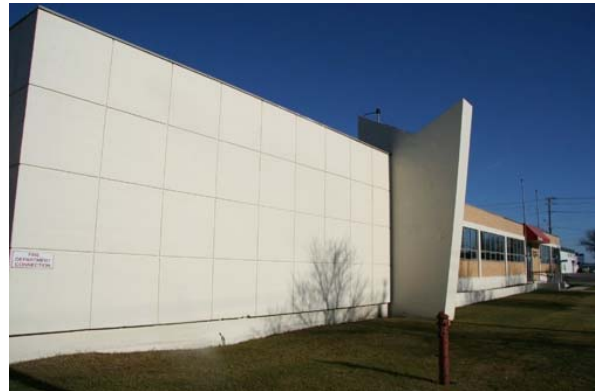
Atlas Graham Building, 1725 Sargent Avenue, Winnipeg
