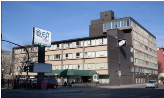
Former Brittany Inn, 1958. 367 Ellice Avenue, Winnipeg
