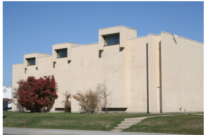
Masonic Temple, 1969. Osborne Junction, Winnipeg.
