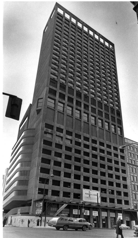
Radisson Hotel, Winnipeg, Number Ten Architectural Group, 1969
