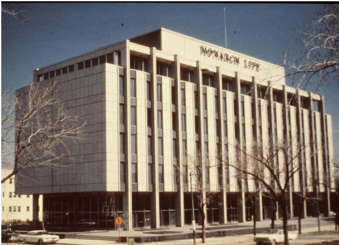
James Donahue, for Smith, Carter, Katelnikoff and Searle, Monarch Life/Worker's Compensation Building, Winnipeg, 1959-63 ( currently being re clad )
