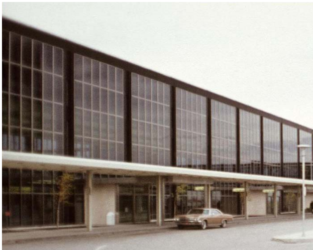
Richardson International Airport, Main Terminal, Green, Blankstein and Russell, 1964 ( now being demolished )
